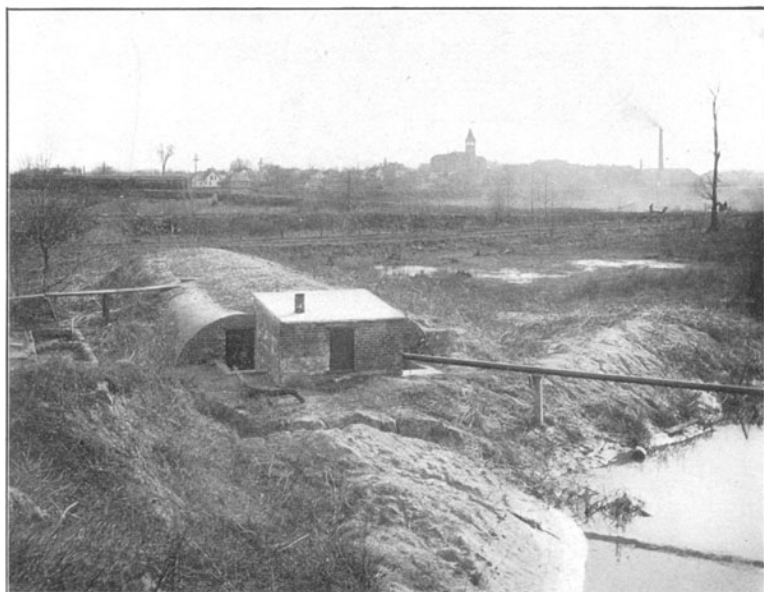
FIG. 4. SEPTIC TANK, URBANA, ILLINOIS, Exterior.
