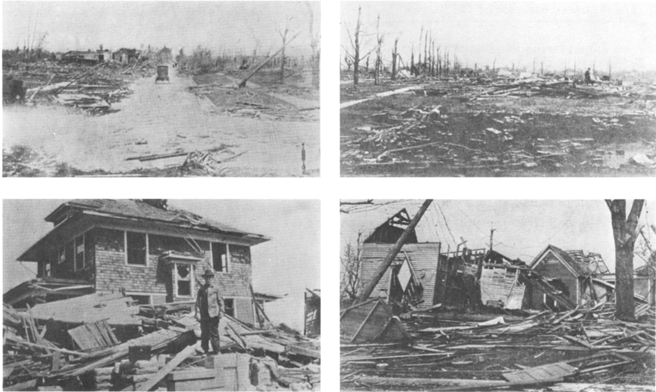
Figure 21. Damage scenes in Mattoon 26 May 1917
