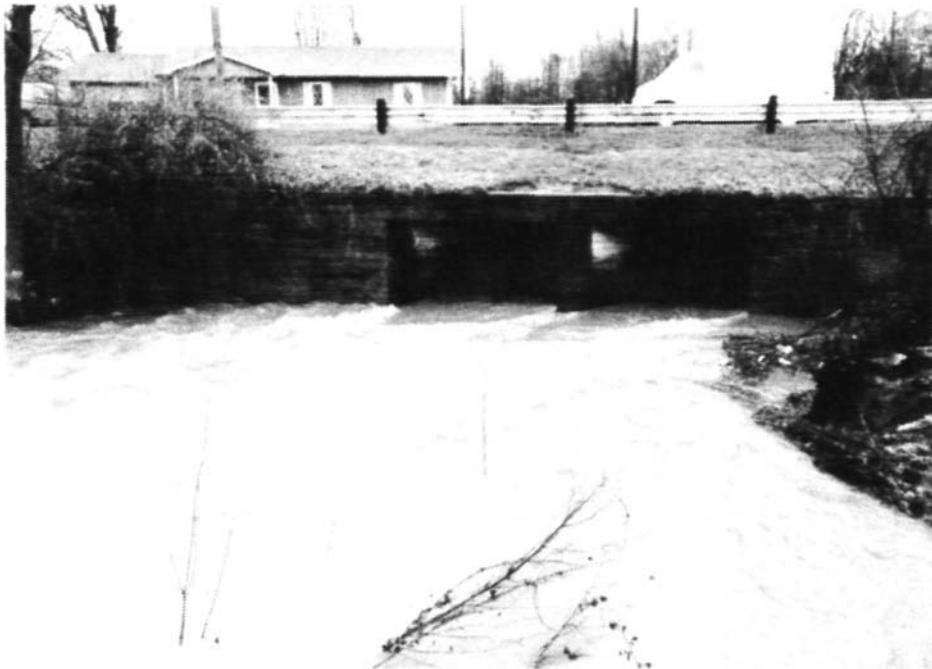
Figure 19. Water exiting Miller City Road box culvert
