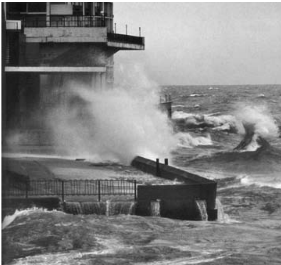
Fig. 2-5. The major increase in the level of Lake Michigan brought high waters and damages to shoreline properties like this building in Chicago, once 1,000 feet from the shoreline.
