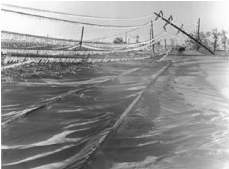
Fig. 6-4. Heavy snows and ice storms in Ohio downed power lines and blocked a rural road.
