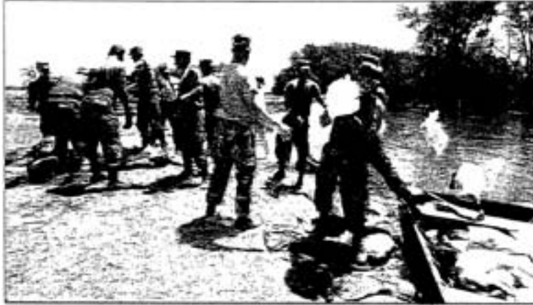
National Guardsmen relay sandbags for use in reinforcing the Big Swan Levee near Winchester. The Illinois River levee, along with the neighboring Scott County Levee, were under watch last week, even as floodwaters started to fall. See more on flooding problems inside. (Photo by Ken Koshian)
