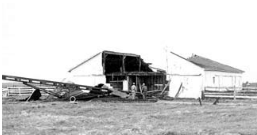
Fig. 4-6. Rural farm buildings in Illinois were damaged by high winds from a June 1990 storm.
