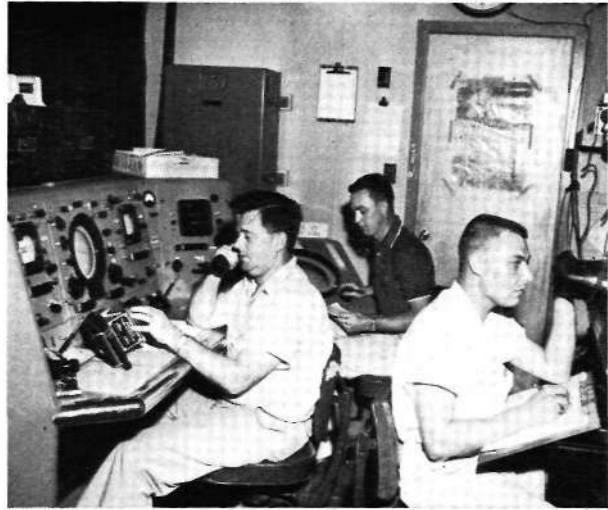
Radar is newest tool used to study rainfall
