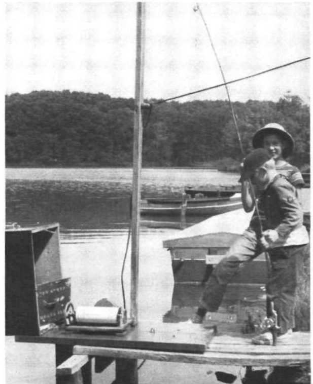
Water-level recorder measures amount of water that a reservoir contains
