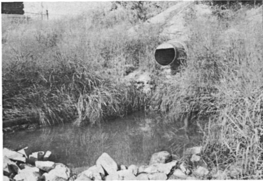
Figure 11. Outlet of Hi-line
